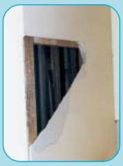
Asbestos insulation board (AIB)
