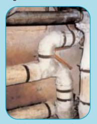
Asbestos pipe lagging
