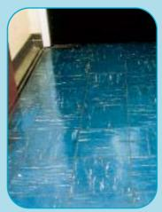
Asbestos-containing floor tiles
